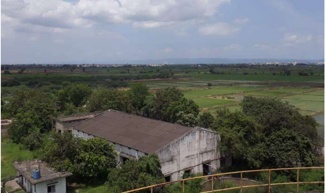
Green belt developed near by Pump House area 2 acres
